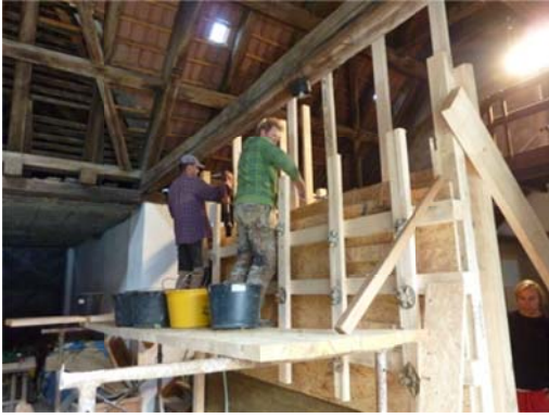
Picture 7: Moving the formwork
