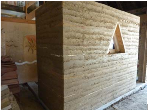
Picture 8: We soon reached the planned height and 4.6 cbm of self-built rammed earth mixed
