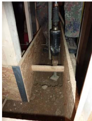
Picture 6: Material compacted with pneumatic rammers
