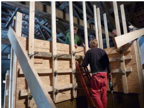
Picture 5: Construction of a pressure-resistant formwork
