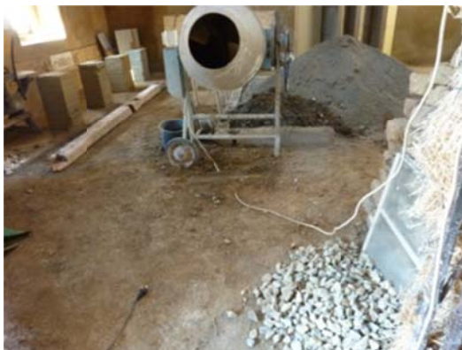
Picture 2: Material mixing with small stones and water
